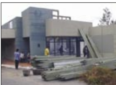
The demolition phase
