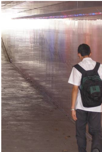
Below: Inside the upgraded Doncaster Hill Pedestrian Underpass.
