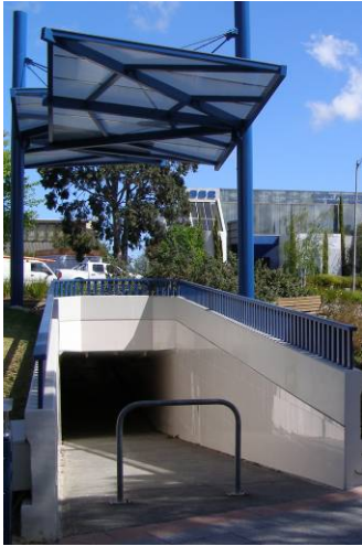
The two newly installed canopy shades, marking the entrance to the Doncaster Hill Pedestrian Underpass
